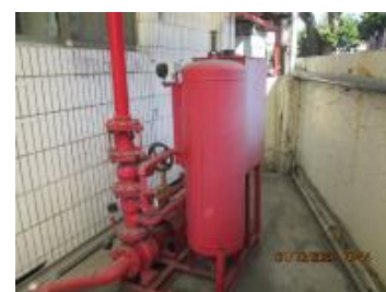
36.Foreign worker dormitory (Fire pump).JPG
